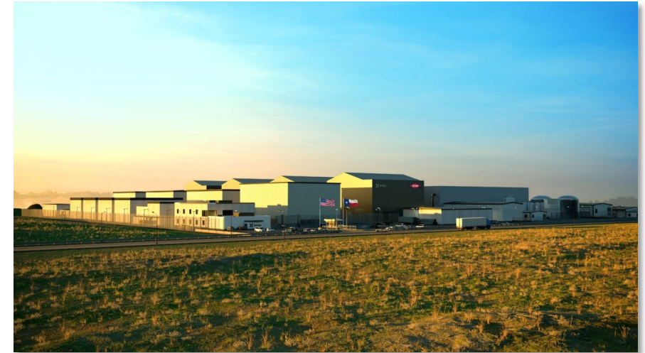
Four-unit Xe-100 plant providing 320MWe and 800MWth to Dow’s Seadrift facility on Texas Gulf Coast
